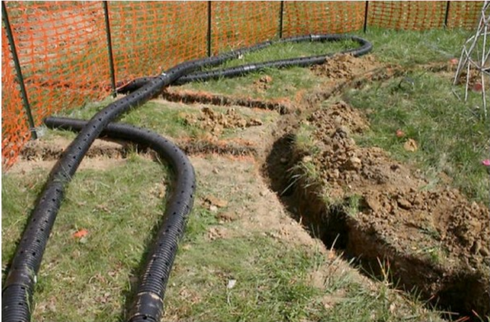
Groundwater recharge in trenches. Source: BATES (2004)
